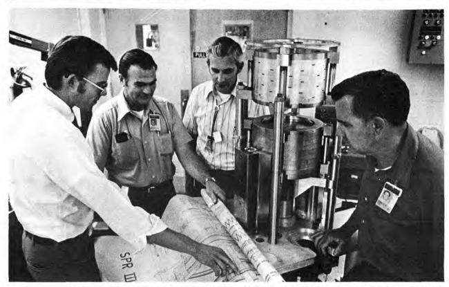
NEW SPR III pulsed reactor is now undergoing mechanical testing in Area V. The reactor with dummy fuel elements — circular configurations at top of the device — is examined by (I to r) Ted Schmidt (5221), John Snyder (5221), John Reuscher (5221) and Don Cox (5222). Test cavity for components and systems is surrounded by circular fuel elements.
